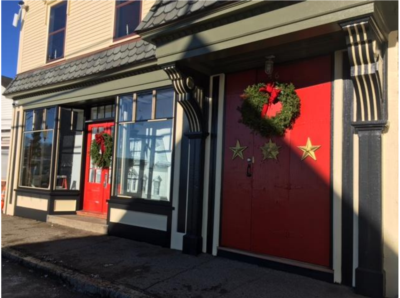
New storefront windows on the Star of Hope building in Vinalhaven
