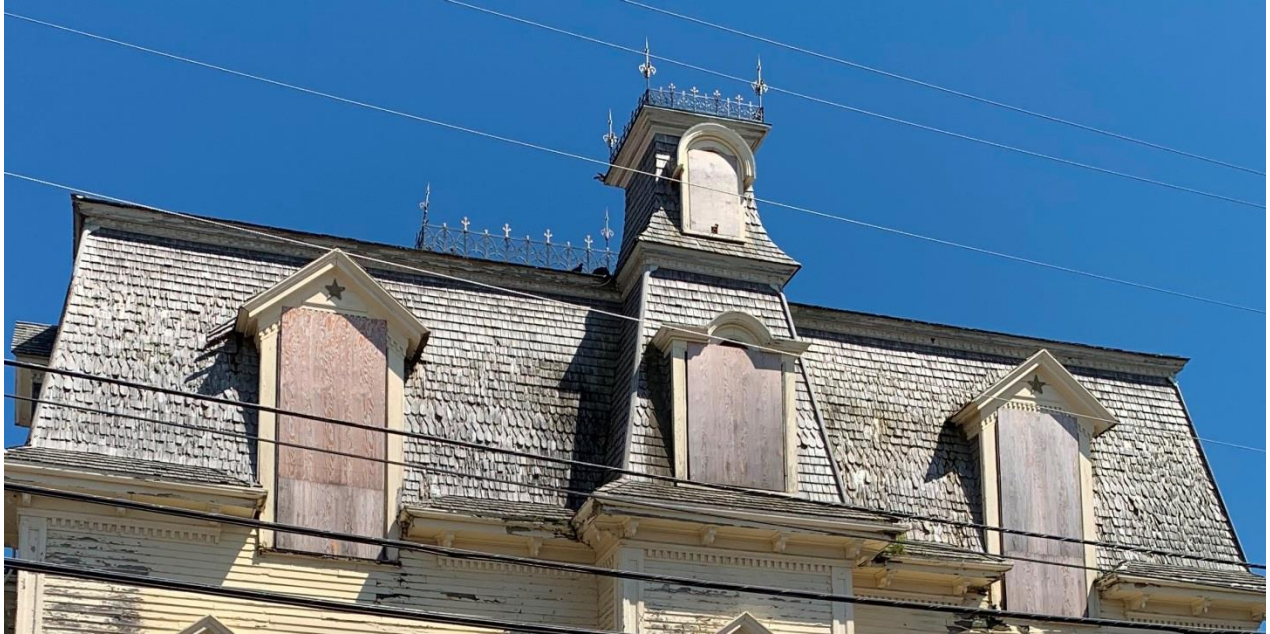
Building Stabilization Efforts Continue on this Historic Landmark
